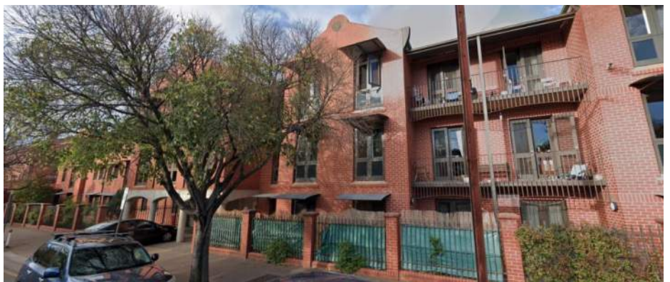
Figure 9: c1990 St Marks dormitory building. Source: Google Streets
