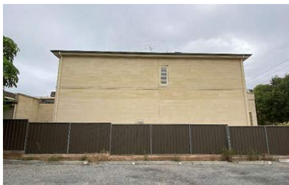
90 Kermode Street (east)
