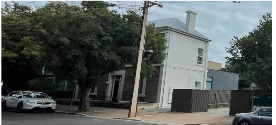
Figure 5: Local Heritage listed two storey residence, 98 Kermode Street North Adelaide.
