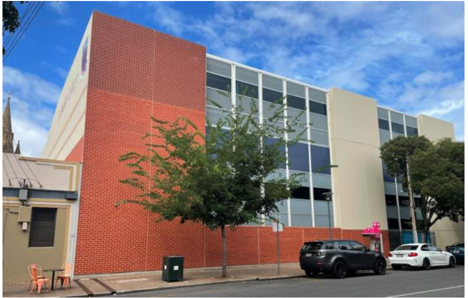
Figure 13: Multideck carpark, 73 Kermode Street
