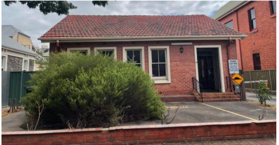
Figure 10: Small office, 78 Kermode Street.
