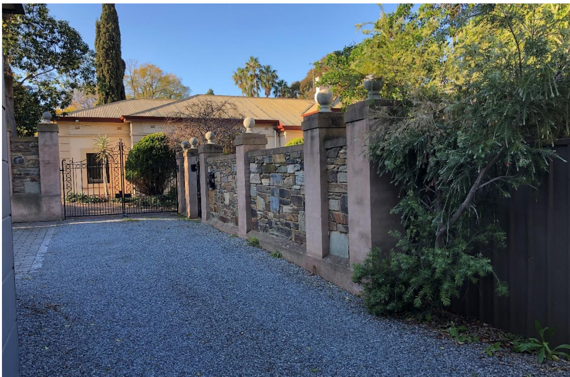
View to the existing wall on the subject site boundary, facing north east from within the right of way
